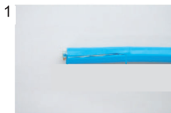
1 Expose inner vinyl sheath.
